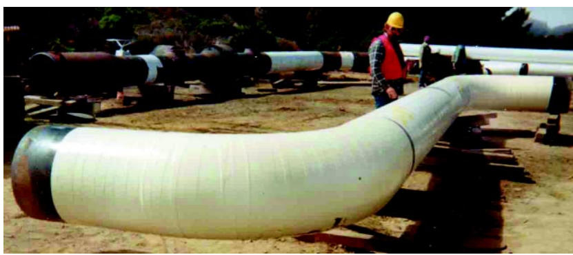
(Left) Brush application of coal tar coating. (Right) Rubberized bitumen tape applied to steel pipe.
