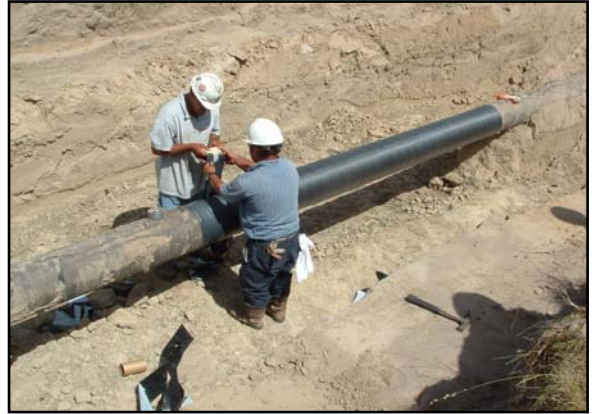
INSTALLING OUTERWRAP
