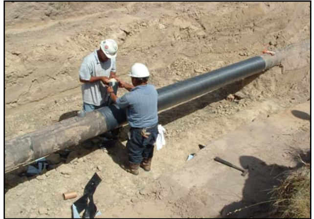
INSTALLING OUTERWRAP
