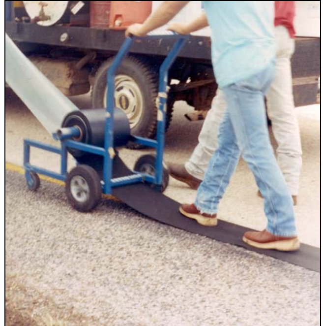
Parking Lots, Pavement Joint & Crack Applications
