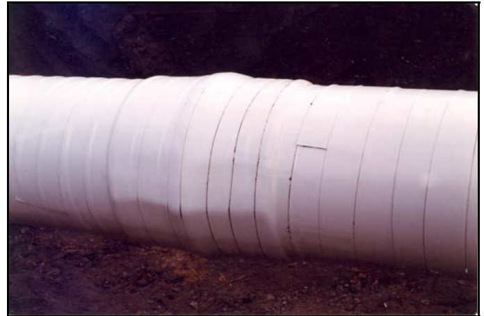
600 Series Coating applied on a rehabilitation project.
