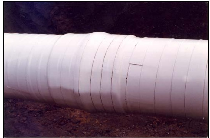
600 Series Coating applied on a rehabilitation project.
