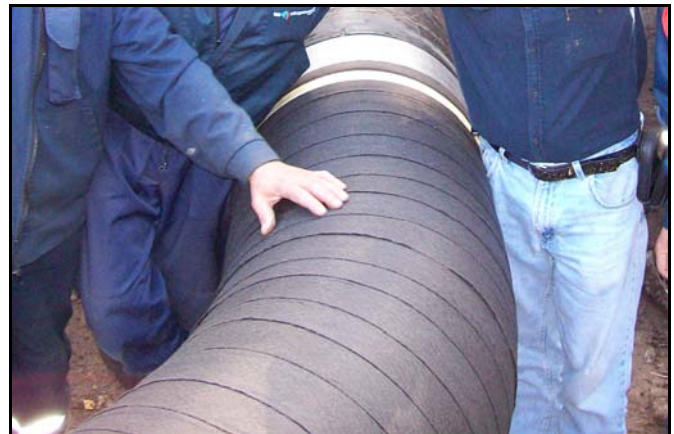
The use of POLYGUARD SP6 OUTERWRAP is also advised for resistance to soil stress.
