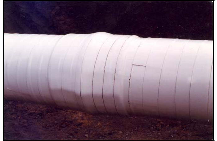
600 Series Coating applied on a rehabilitation project.
