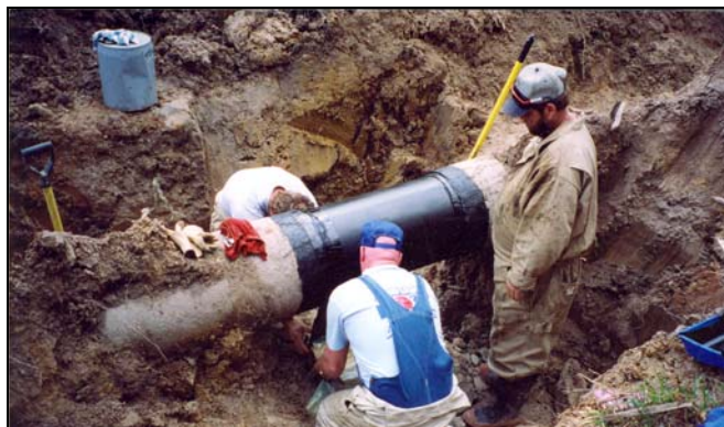
606 Filler Tape can fill irregular transition areas, thus avoiding gaps and voids under the coating.
