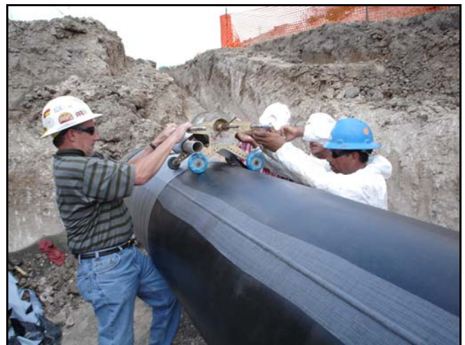
Application by machine permits the coating to be installed under higher tensions. This aids resistance to soil stress.
