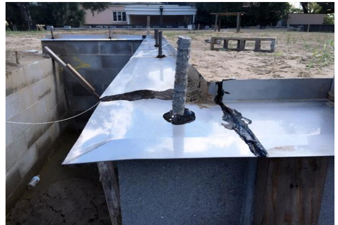
Termite shield sealed with TERM Sealant - New Orleans home
