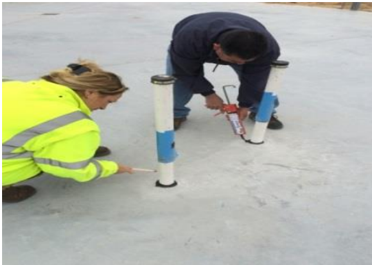
Sealing penetrations at an Austin bank
