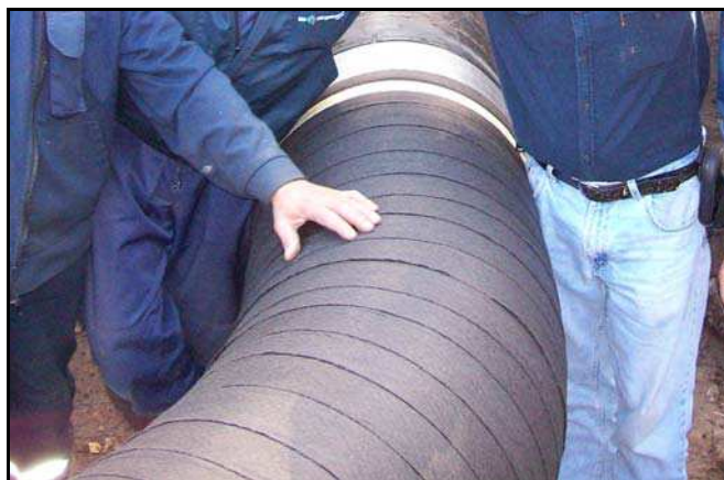
The use of POLYGUARD SP6 OUTERWRAP is also advised for resistance to soil stress.
