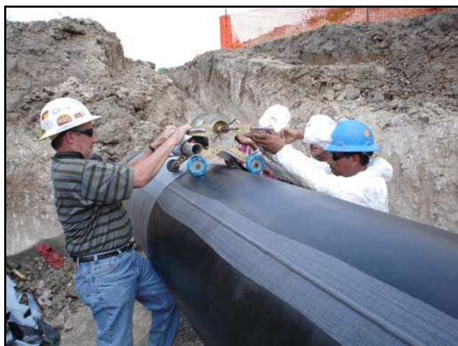
Application by machine permits the coating to be installed under higher tensions. This aids resistance to soil stress.
