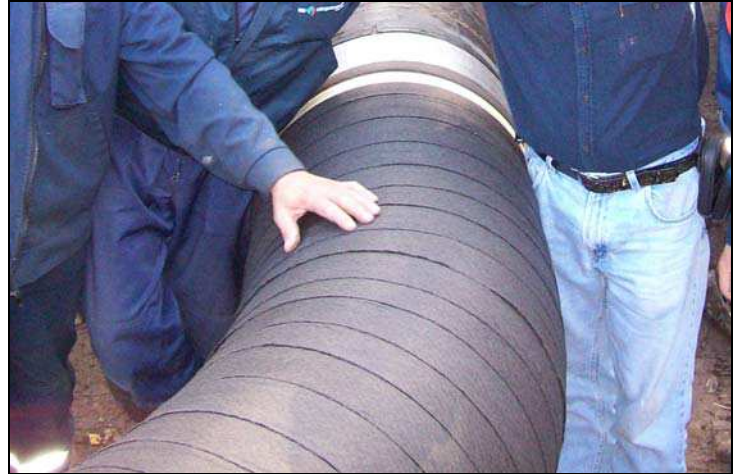
SP-6™ will reduce the deformation of corrosion coating systems caused by soil stress. It acts as a slip plane to relieve soil stress.
