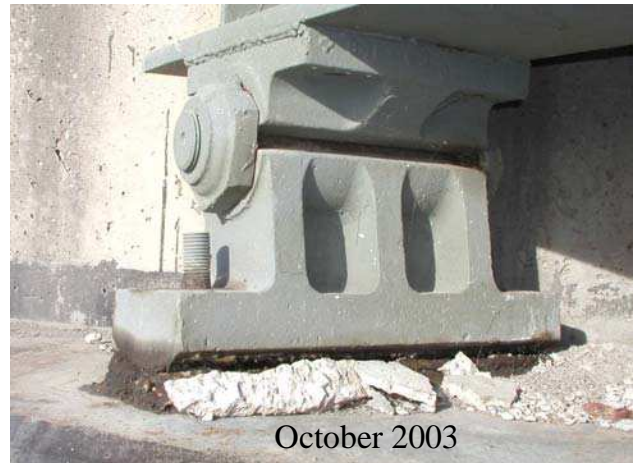
Figure 7 – Rocker Assembly Inspection – October 2003
