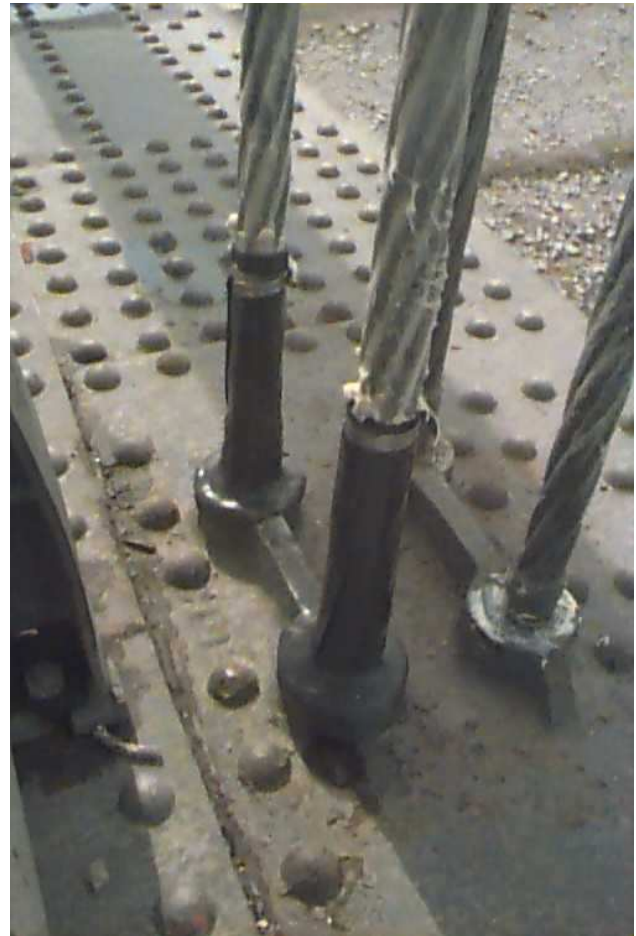
Figure 10 – Bridge Stay Finished Application – March 2004
