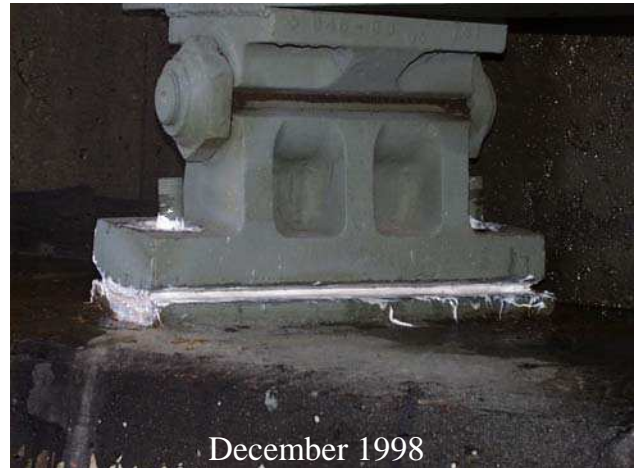
Figure 5 – Rocker Assembly After Gel Application - December 1998
