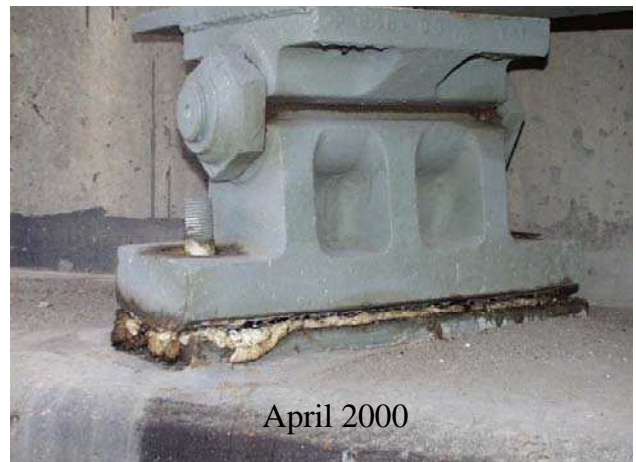
Figure 6 – Rocker Assembly Inspection – April 2000
