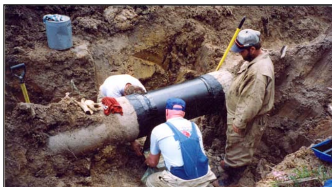
606 Filler Compound can fill irregular transition areas, thus avoiding gaps and voids under the coating.
