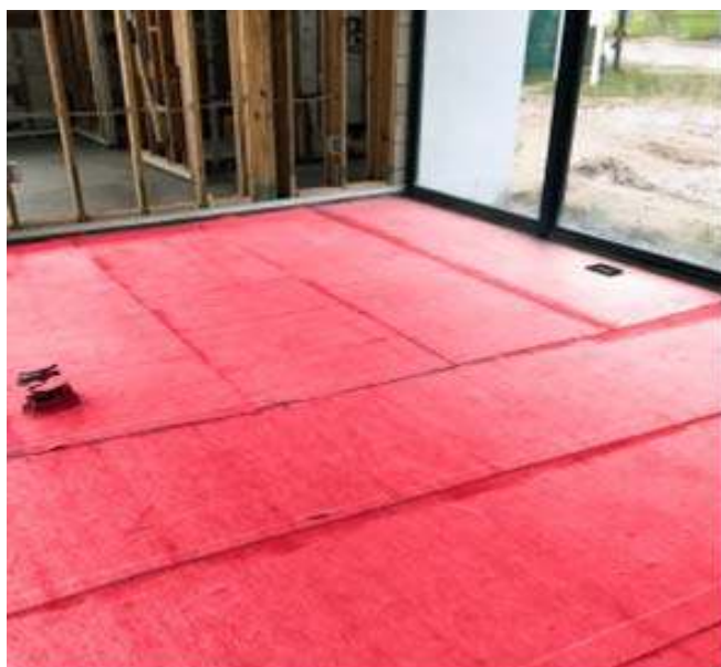
TERM® Tile Underlayment|Termite Barrier installed in The New American Home – 2017 , built by NAHB in Orlando, FL
