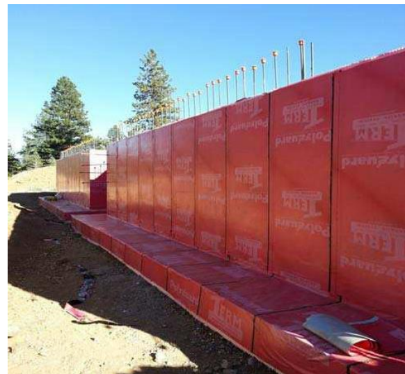
1 - ICF Foundation - Verdi, CA
