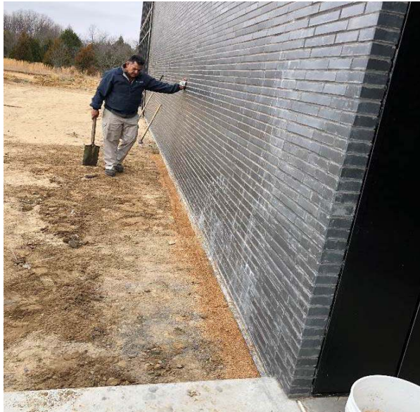
TERM Particle Barrier installation – Oklahoma medical center
