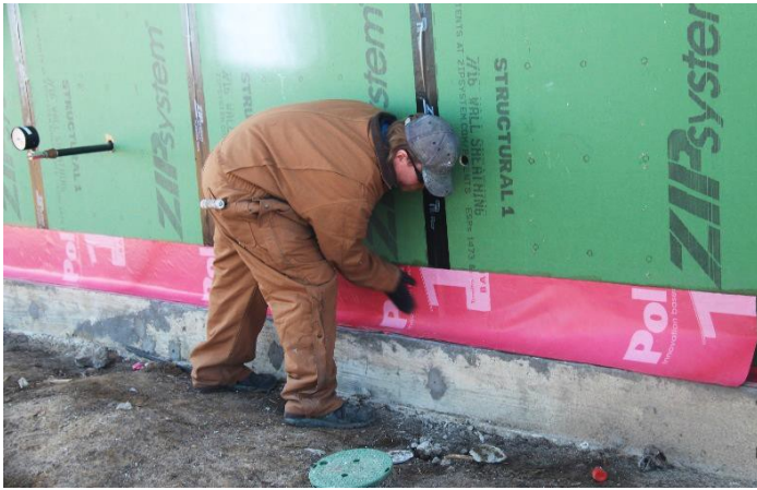
TERM Flashing|Termite Barrier installed on a residence in Ennis, TX
