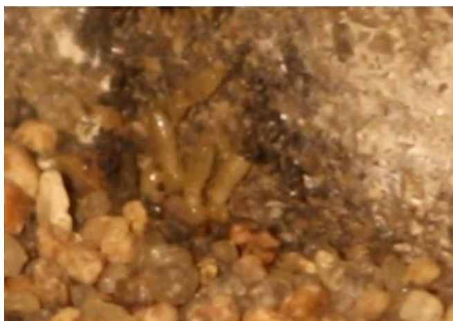
TERM Particle Barrier installed around exposed perimeter concrete at an Oklahoma hospital
