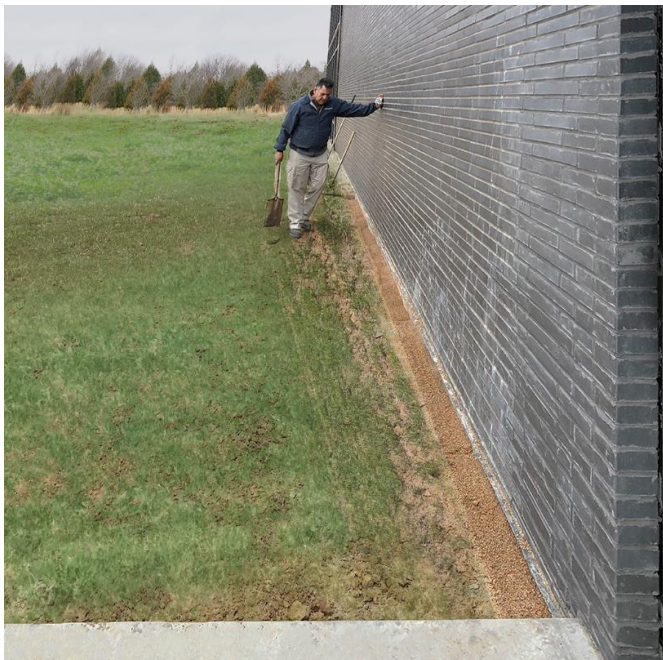
TERM Particle Barrier installed around exposed perimeter concrete at an Oklahoma hospital
