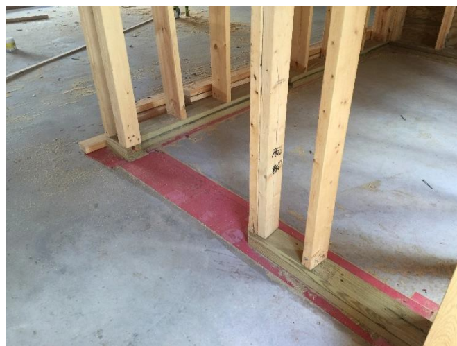
Interior sill – Orlando, FL
