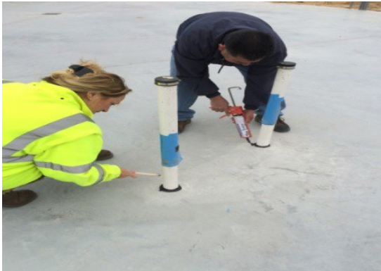
Sealing penetrations at an Austin bank
