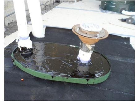
**Gas Vapor Protection** For full gas vapor protection all pipes must be wrapped using the **TERM UVR Barrier Tape** and secured to the pipe with a screw clamp.
