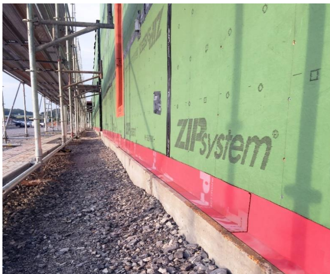
TERM Flashing|Termite Barrier installed on an Oklahoma hospital
