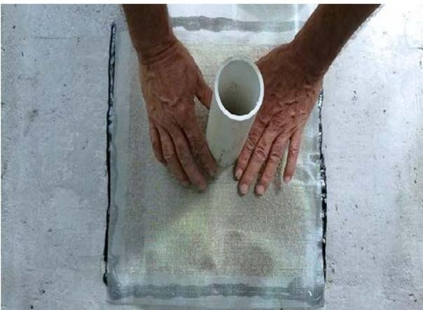
**Step 7:** With the wire mesh section in place over the first layer of sealant, place a second 3/4" bead of sealant on top of the edge of the wire mesh making sure that the sharp edges of the wire mesh are covered with sealant
