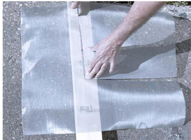
**Step 4:** Cut an opening in the *TERM Micromesh 02* for the penetration. This is done by positioning the wire mesh section over the cavity and the penetration at a point where the 2" border will be maintained all around the cavity. Then use a rubber mallet or hand pressure to create an impression of the top of the penetration in the wire mesh. Now cut a hole in the wire mesh just wide enough for the wire mesh to fit snugly over the penetration.
