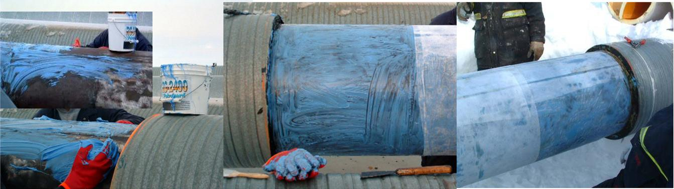
**RG-2400® AK is designed to be installed on hot pipes (above 100°F) it is difficult to spread on a cold surface due to its thicker viscosity. For ambient of cold pipe application, use RG-2400 LT.**
