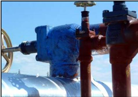
**RG-2400<sup>®</sup> LT** helps prevent corrosion from occurring, and it also helps stop existing corrosion from advancing. It requires minimal surface preparation (wire brush off the scale). In addition, **RG-2400 LT** can help prevent stainless steel and copper stress crack corrosion under insulation.
